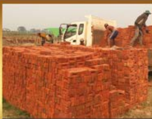
The bricks for all the exterior walls are delivered.
