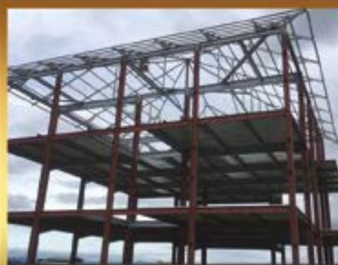
The Legacy building takes shape.
